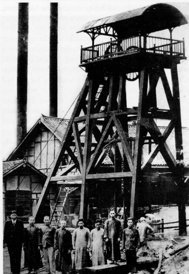
Original headgear from when the mine opened in 1938
